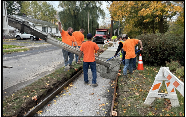
DPW staff installing new 5 ft. wide sidewalks on Clark St.
